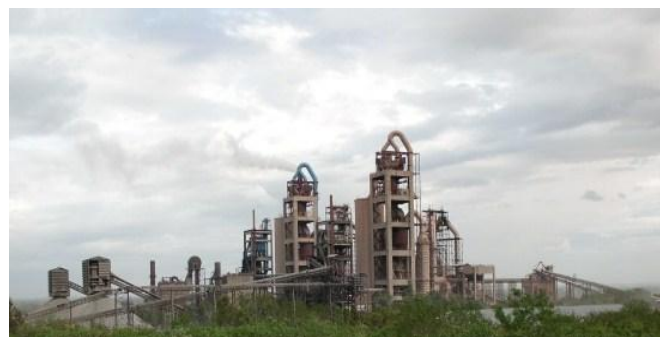
India Cements Ltd. automated its Malkapur, India, cement plant with Honeywell's MasterLogic PLC and Experion solution.
